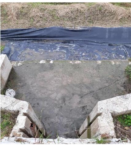
A photograph of a concrete gate structure for the lagoon. The gate is partially submerged in water. Above the gate, there is a black plastic geomembrane covering the ground.                     |
